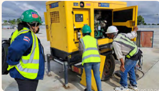
Site Safety Inspection
